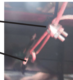
Cable clamp and ridge cable loop
