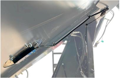
Route the wire from the moisture sensor up the bracing using the wire looms provided as shown in the image to the left. Connect the 9' moisture sensor cable (JM0060736) and connect to the iFarm Cart box.
